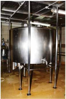
The milk tank must be installed in such a way that a food-graded milk pipe can be connected from the delivery vehicle to the milk tank.
